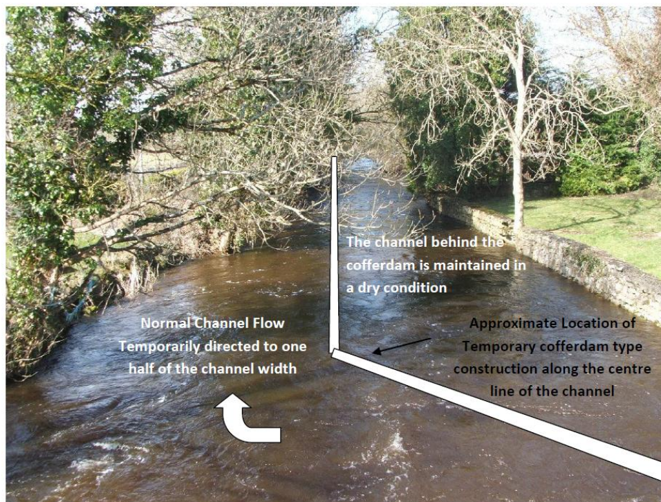
Figure 3-8 – Proposed Works Channel Works in the vicinity of Craughwell Village and sketch of cofferdam location
