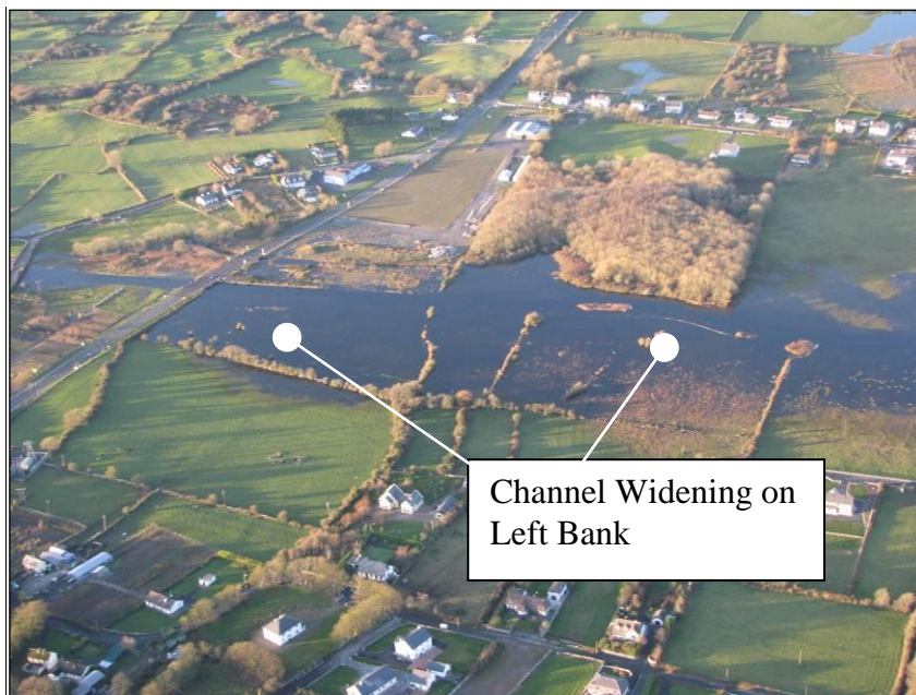
Photograph No. 29 – Location of Channel Works downstream of Killeely Beg Bridge
