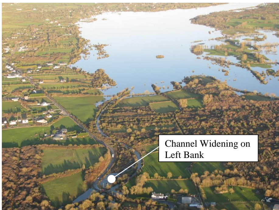
Photograph No. 27 – Location of Channel Works upstream of Rinn Bridge
